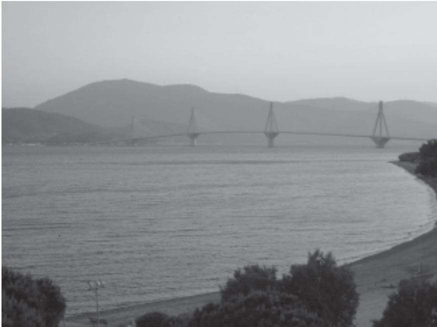
Bridge connecting Northern Greece to Southern Greece (Peloponnesus)
