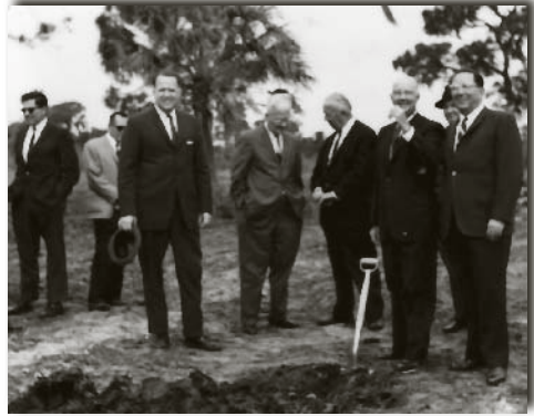
Ground breaking - Mayor Turner on right, 1966
